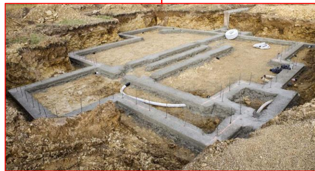
4. Build from the Foundations Up
